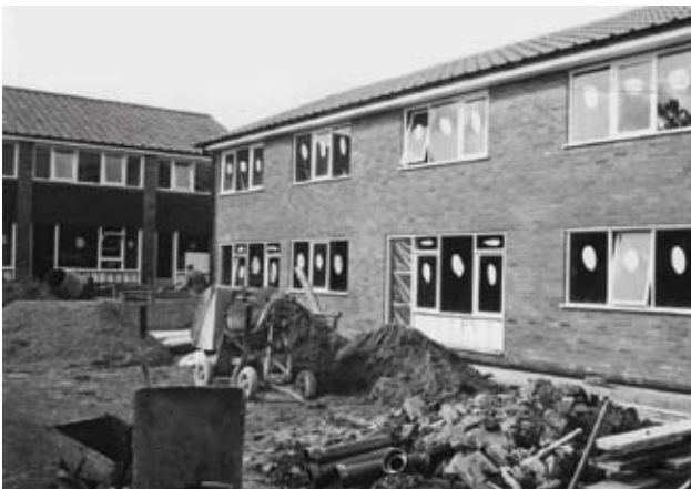
East Borough Flat in the final stages of construction in 1966
