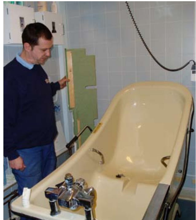
Plumbing repairs in progress
