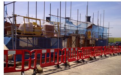
Cambridge Court Phase Two underway
