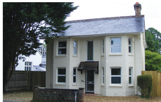
Front view of the other newly developed property in Lymington Road
