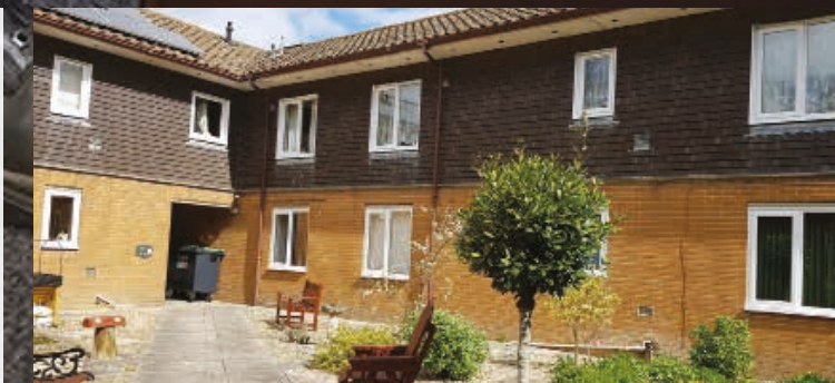
New double glazing installed at Butts Mead House, Shaftesbury
